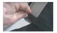
Work around the support bar by moving it back and forth a little if installing the UltraWeave fabric into grip rails.
