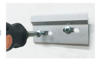
First, attach the two brackets to the wall. You an slide the frame so you are free to place the brackets as much as 20-40cm from the corners.
